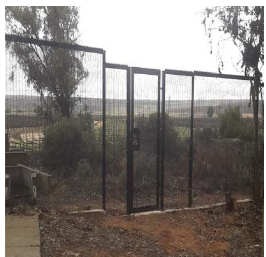
Fence and automated gates at the Koekenaap cultural facility.
